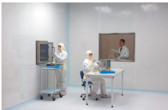
BioSafe interior FRP panels: Class A fiberglass-reinforced plastic (FRP) panels provide a 100% sealed, fire-rated, ISO 5-compatible enclosure
